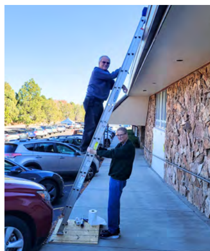
repairing a leak in the gutter
